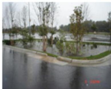
A rain garden absorbs parking lot runoff at Northlake Mall.
